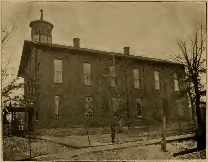
COURT HOUSE AT OAKLAND.
